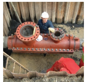
Installation of double branch Grouted tee
