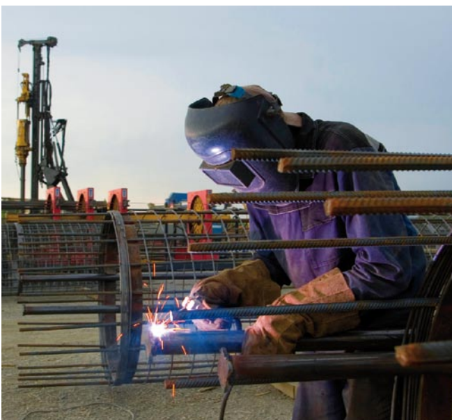
Welding of reinforcement steel
