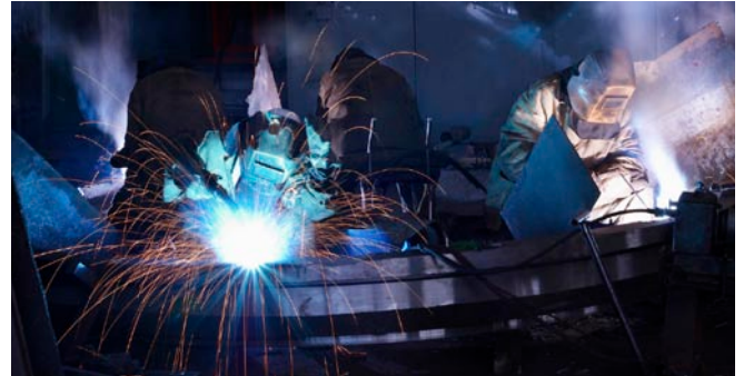
The more efficient solution: on-site welder qualification test for a group of welders
