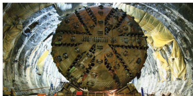
Tunnelling machines: technically challenging due to longer, deeper tunnels, geological conditions, etc.
