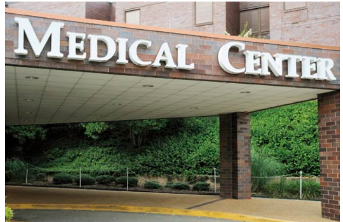
Hospitals can also be equipped with a GL inspected and certified hyperbaric medical treatment chamber
