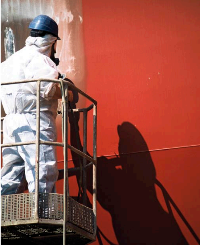
Corrosion protection – still manual work
