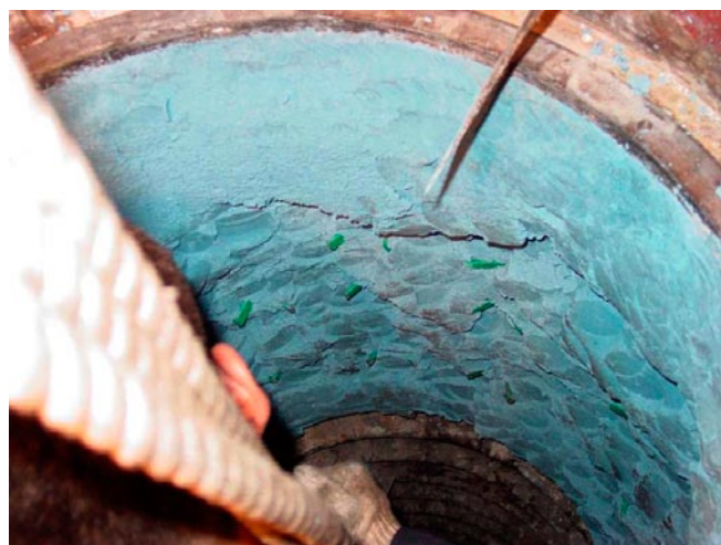
Installation of new brickwork
