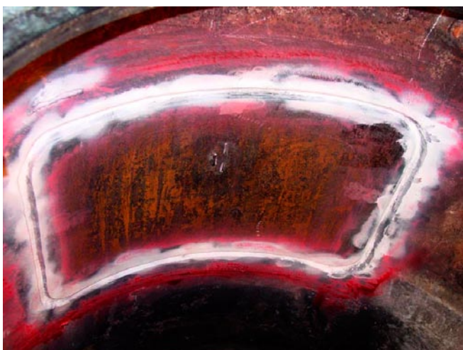
Replacement of defective material (approved repair procedure)
