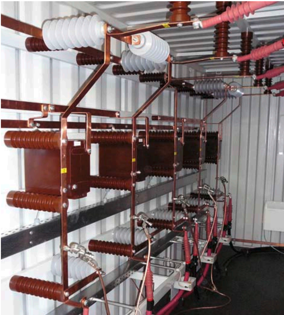
Measurement transducer installed in the WINDTEST equipment.
