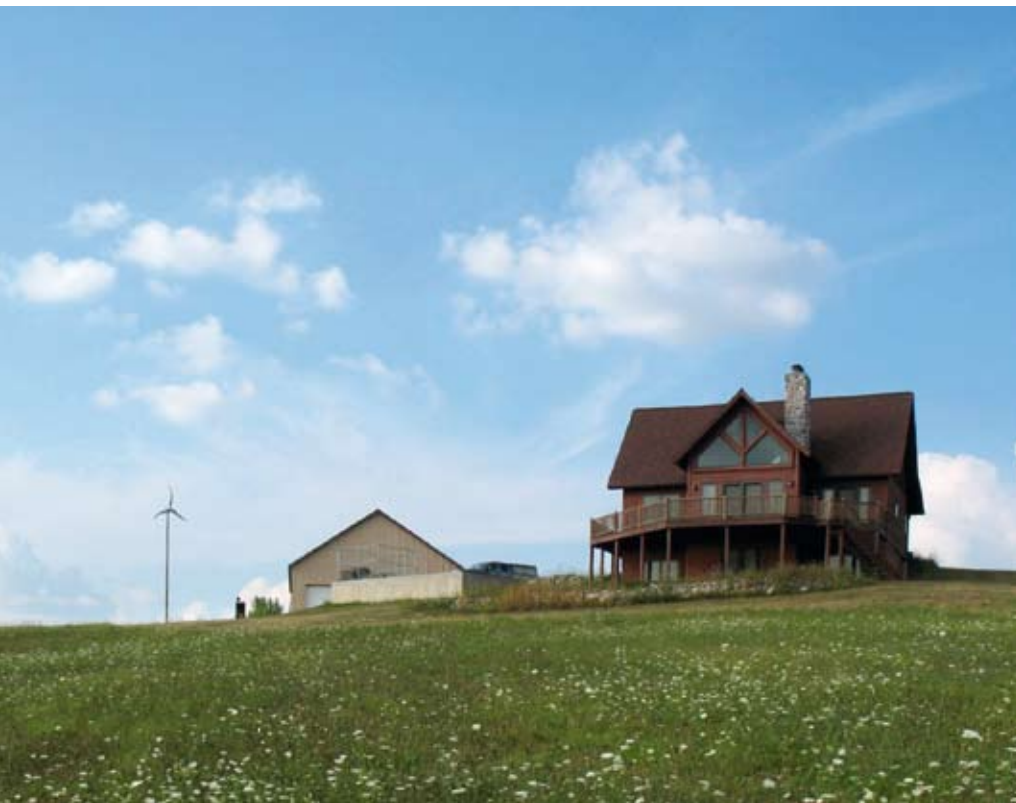
This small wind turbine supplies an isolated house in the US with electricity.
