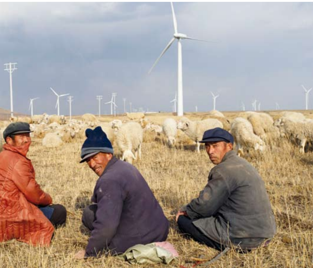
The Shiren wind farm near Shangyi in Hebei province.
